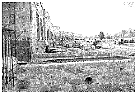
Building Entry Site walls
